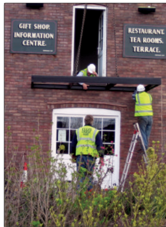
The balcony being erected against The Wharf House in 2011.
