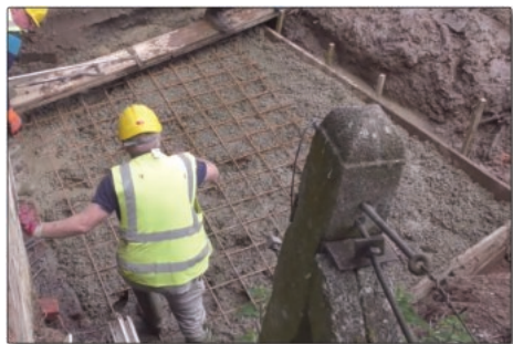
The Malswick team, led by Robert Heigham, prepared the chamber base at the upstream end of the larger culvert and started laying the first few courses of blocks.
