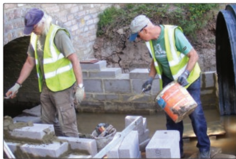
The Malswick team, led by Robert Heigham, prepared the chamber base at the upstream end of the larger culvert and started laying the first few courses of blocks.
