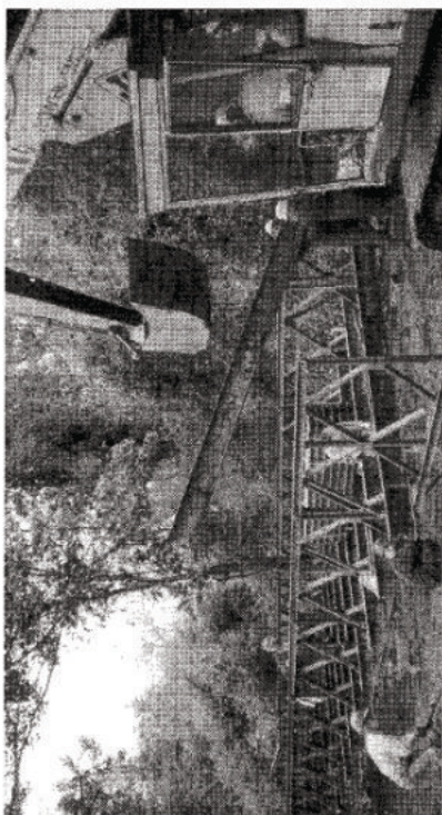
ABOVE: The last cross-beam is carefully lowered into position. BELOW: The Bridge reaches the far side - 3 more bays of "launch nose" to come beyond the rollers. These are removed to leave a 5 bay Bridge. RIGHT: The first section of decking is put into position.
