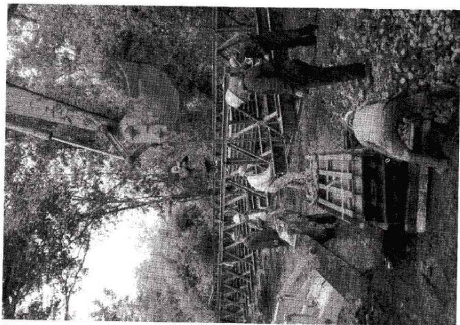
LEFT: The Bridge slowly advances above the dilapidated aqueduct. RIGHT & BELOW: The last section is placed in position, together with stacks of decking on the Bridge to act as counterweights, before the last push.
