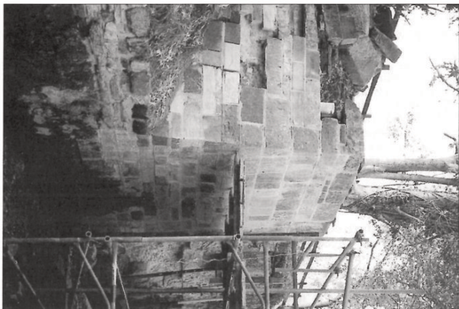
Work on the downstream end of House Lock. Oxenhill is beginning to turn a crumbling ruin into a very attractive – and soundly built – lock. Before long the lock chamber itself will become the focus of attention.
