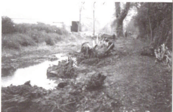
◆ Above and below: The main task is removing tree roots from the Canal channel and clearing the tow path in preparation for pedestrians and cyclists.
