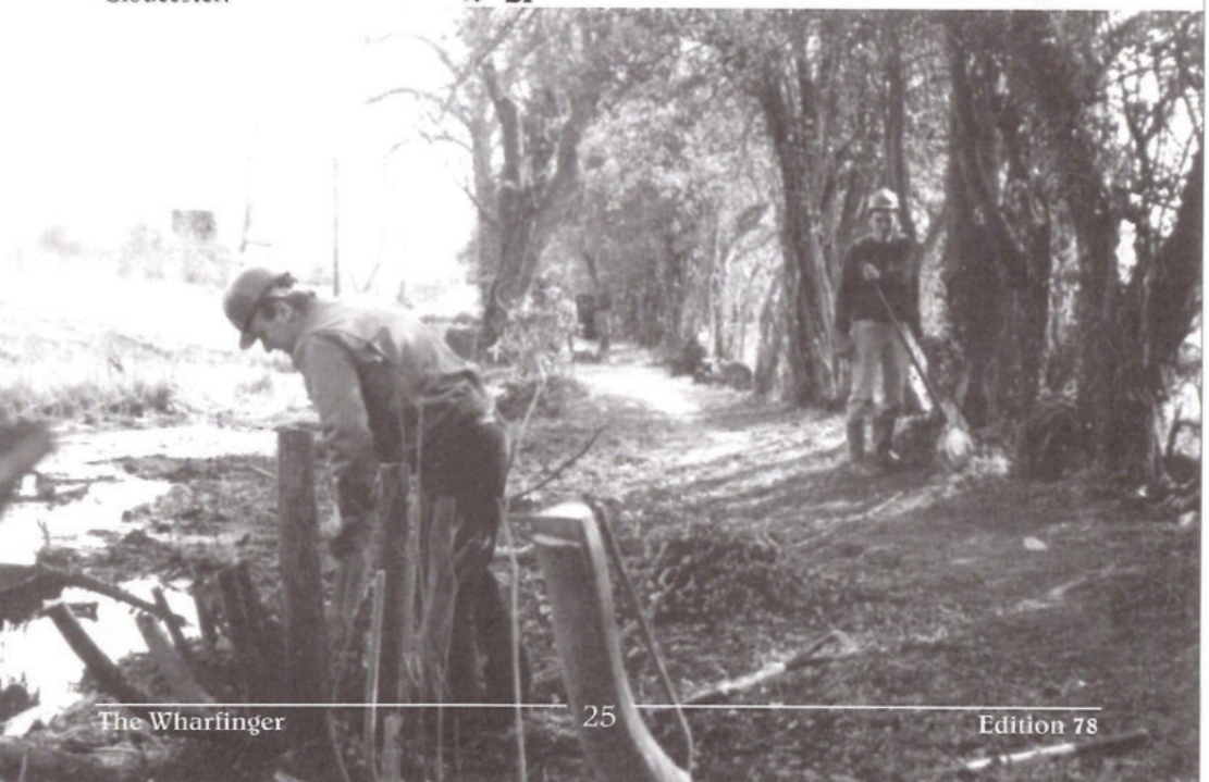
◆ Above and below: The main task is removing tree roots from the Canal channel and clearing the tow path in preparation for pedestrians and cyclists.
