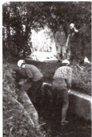
Top left: Alan Flexman gets to the root of the problem with an axe. Bottom left: the foundations for a culvert headwall are begun. Below: Tree roots are winched out of the deep mud.
