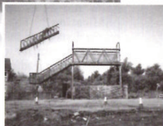
One section of the lower stairs is lifted on to a waiting lorry.
