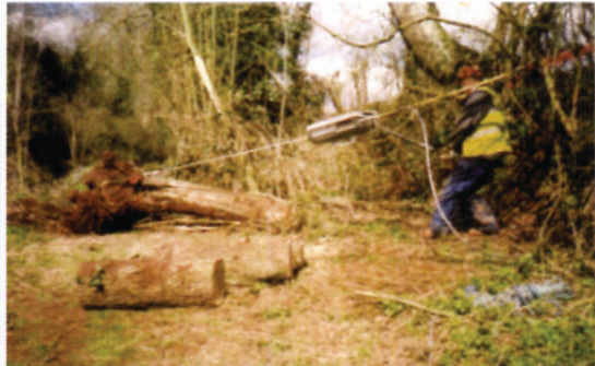
Above: Winching a fallen oak including its roots from the canal corridor.
