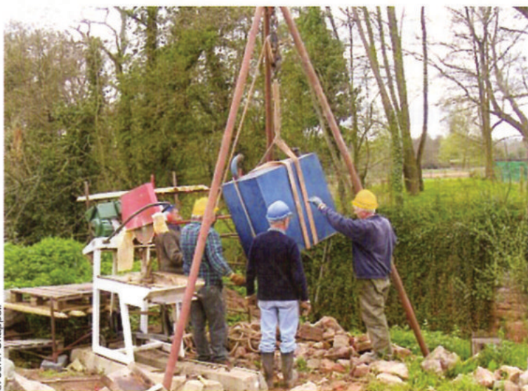
The tank for the water supply to the brick saw is hoisted into position
