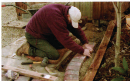
Paul lays the last few edging blocks up to the back gate of THE WHARF HOUSE .
