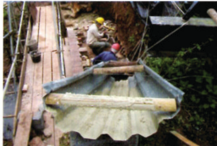
Left: A chute enables materials to reach the aqueduct builders below. Left lower: The area behind the arch is filled in.
