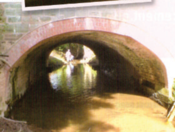
Above: Under the arch showing the join between old and new masonry.
