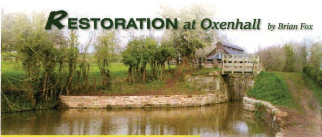
The extended and heightened wing walls to House Lock.
