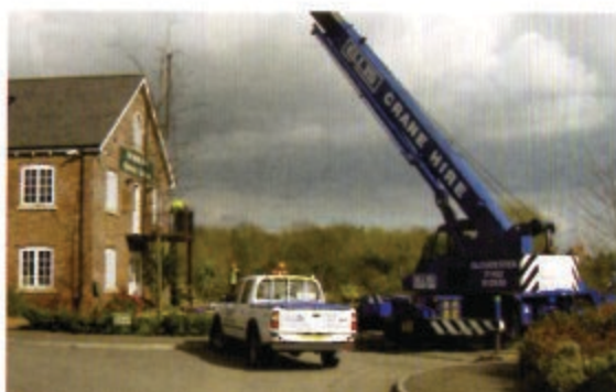
The day of the 'big lift' as the balcony is assembled with the aid of a large crane.
