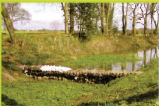
Below: The temporary dam holds back 450 yards of water.
