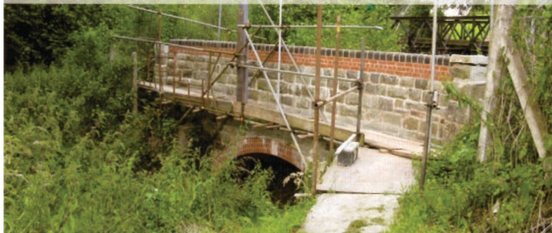
The top coping stones have now been laid to complete one side of the aqueduct.
