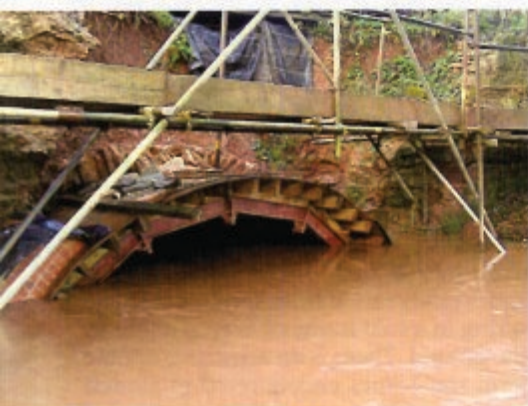
Ell Brook Aqueduct with our steel former in place at the height of the flood.
