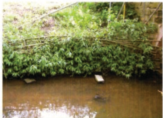
A live willow fence keeps the bank stable adjacent to Ell Brook Aqueduct.
