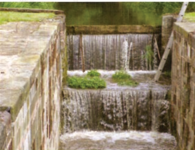
Two stop planks have been removed from the lock.
