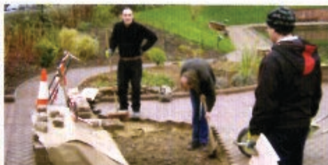
The paviors are being relaid in places where heavy vehicles have caused settlement.
