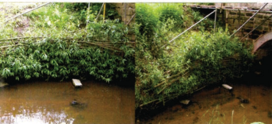
A live willow pile wall keeps the bank stable adjacent to Ell Brook Aqueduct.
