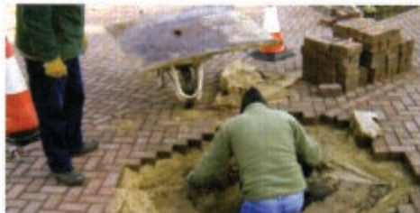
Wilf Jones checks the foundations dug for the drop bollards at the entrance to Over Basin.
