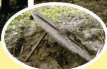
Above: Pivot plate from the old swing bridge.
