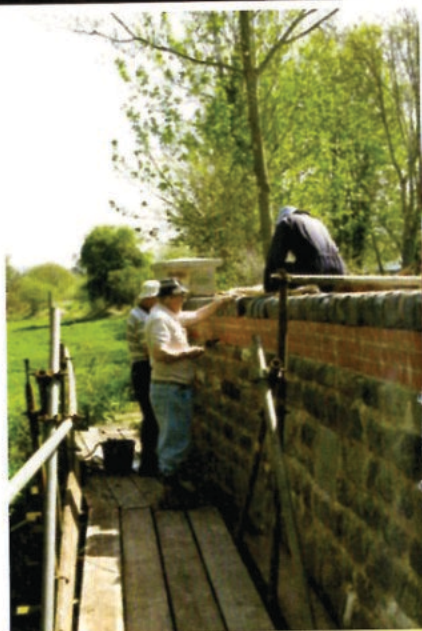
Finishing touches being made to the aqueduct by our team of volunteers. Top photo: Our steel former in place under the aqueduct during restoration.
