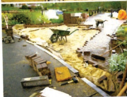
Top: Wilf 'tunes in' whilst 'whacker'ing the sand base.
