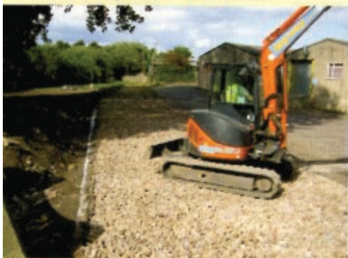
Compacting the hard core.
