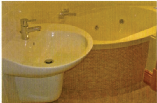
One of the recently fitted smart wash basins.
