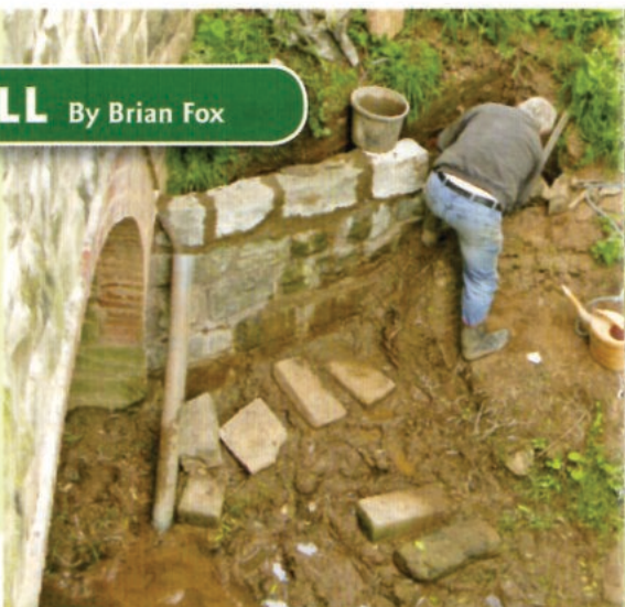
Ian building the wing wall to the Aqueduct.
