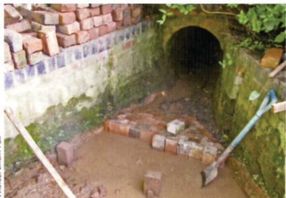
Above and left: Rebuilding the by-weir next to Oxenhall Lock.
