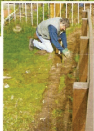
Wilf on his knees (again!) infilling the trench for the cabling.
