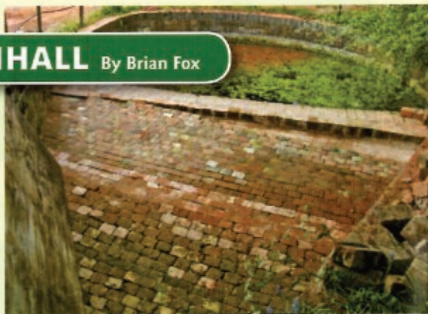
Spillweir nearing completion.
