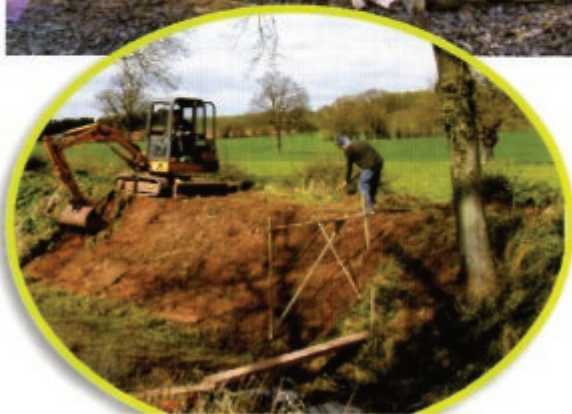
Wild side canal bank profiling starts.
