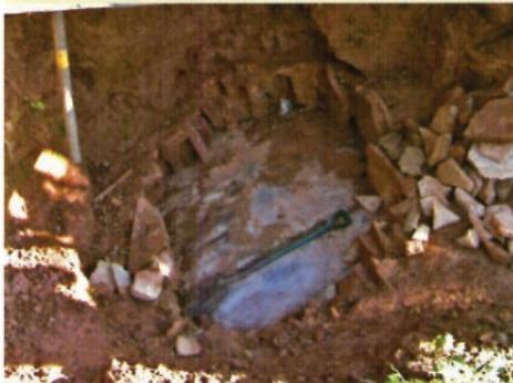
The hole in the top of the aqueduct. The spade in it indicates the large size of the hole.
