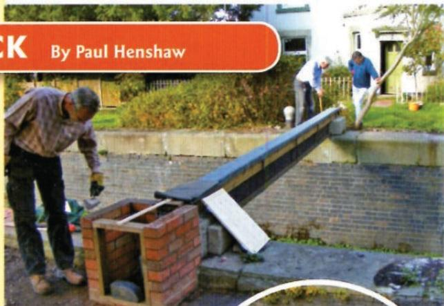
Top: The boxing in of the water supply and the cabinet nearing completion.
