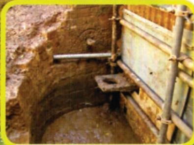
Detail of the offside edge and brick base of the lock chamber.
