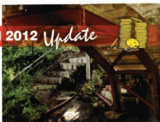
Part of our steel former for restoration of the Ell Brook aqueduct that Fund Members contributed to in 2005.
