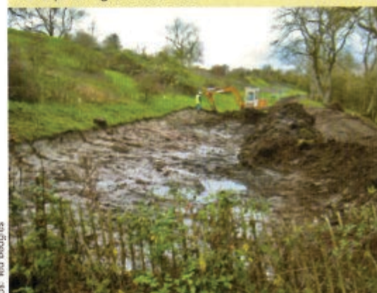
The top soil is stripped back ready for excavation.
