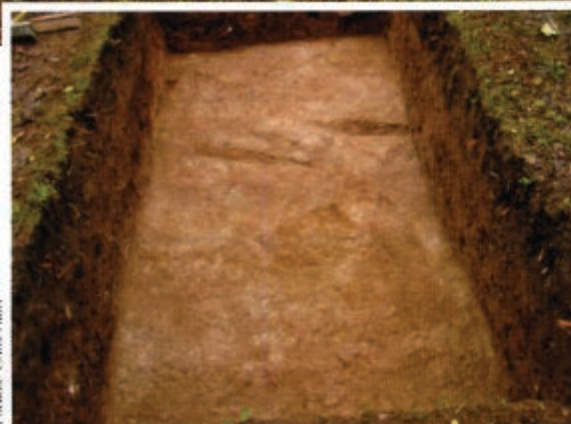
Left: A new lock trench is dug.
