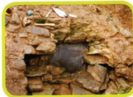
Above: Stumps removed from the culvert portal wing walls.
