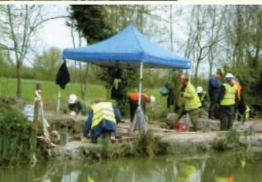
The bricklaying begins on the overflow weir.
