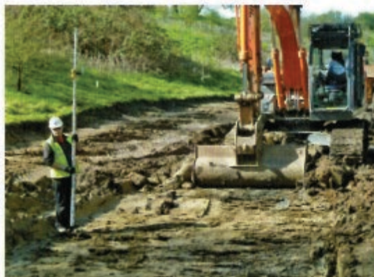
The bed of the canal is levelled.
