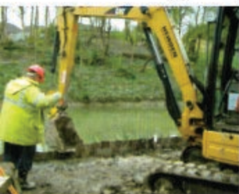
The piling is put in place for the new overflow weir whilst we have the plant on site.
