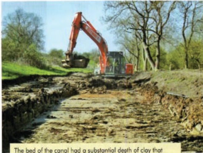
The bed of the canal had a substantial depth of clay that provided the source for constructing the new towpath bank.
