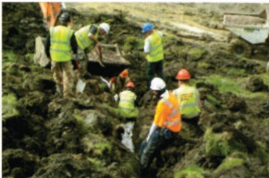
Filling in the French drain by hand.
