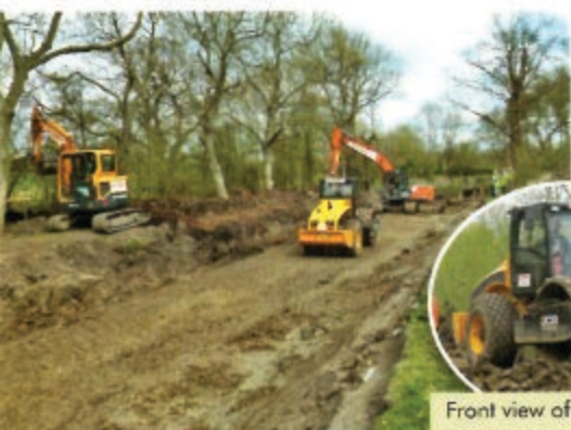
The 13t sheepsfoot roller compacts the clay.
