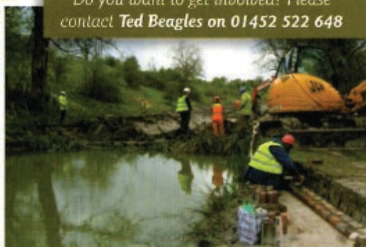
Bricklaying commences for the overflow weir.
