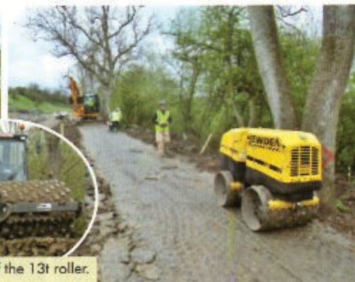
A smaller, remote control version, of the roller.
