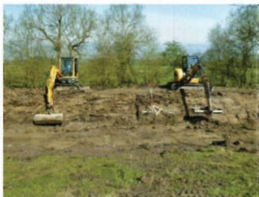
The banks of the towpath are profiled.
