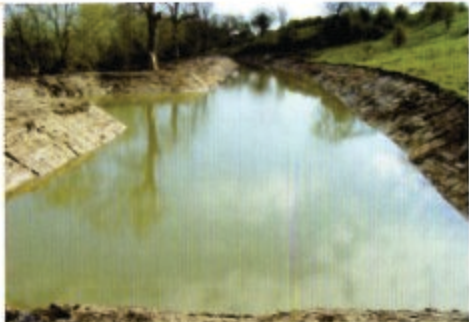
Looking up the new canal from the far end, (winding hole on the left) as the water rises.
