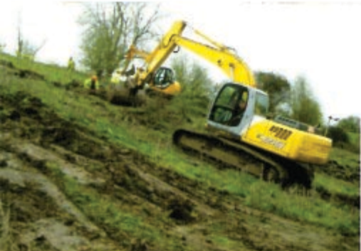
Digging the French drain on the steep slope.
