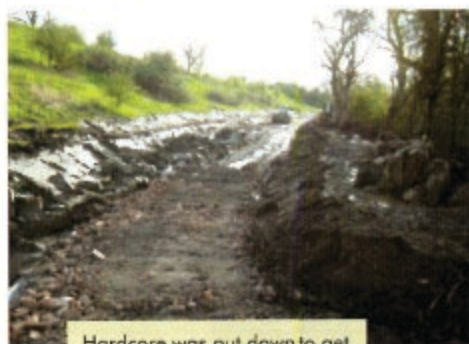
Hardcore was put down to get plant through from the access.
