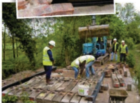
The concrete sleepers are placed.
