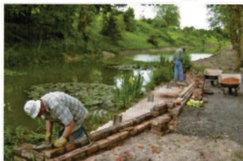
Ivor and Bob building walls of the overflow weir.
