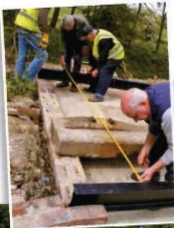
The steel lintels are set in place.
