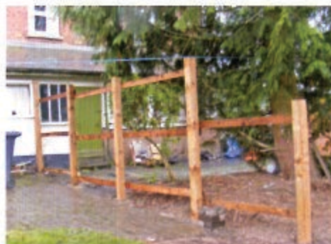
Erecting the fence between the two cottages.
