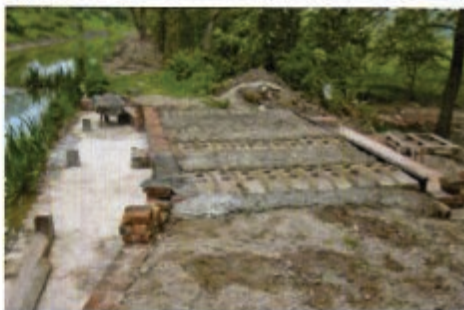
The completed deck prior to surfacing.
