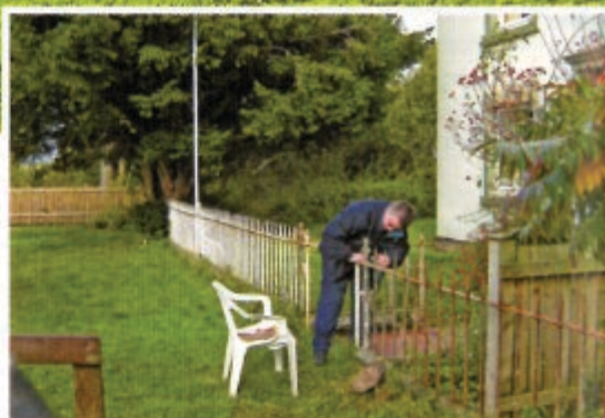
Stripping off the many layers of paint.
