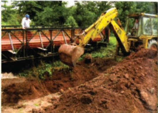
Stripping off the soil ready for the concrete pour.
