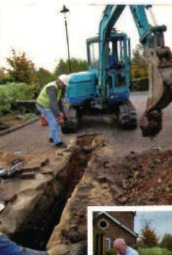
Above: The drainage trench is dug to the bollard.
