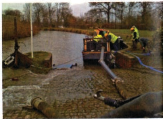
Below and right: Mister Maysey is pumped out with the 6" SPP pump.
