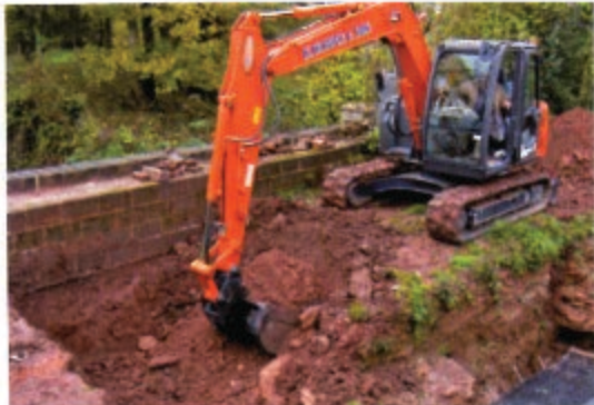
Preparing the ground for laying the concrete membrane over the aqueduct.
