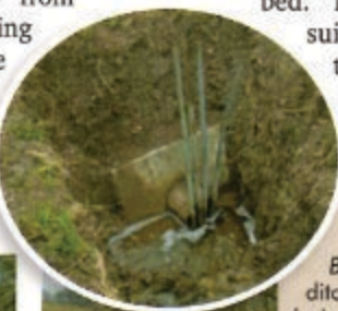
Left: Drain headwall found 4 feet down in adjacent field.
