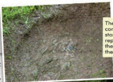
Puddling under way over culvert stonework in the bed of the canal.
