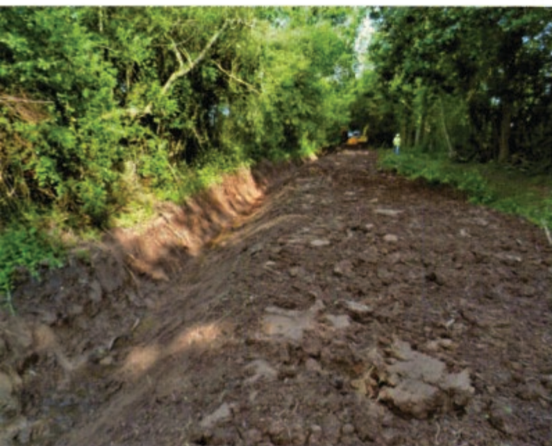
The drainage trench is dug along one side of the canal.
