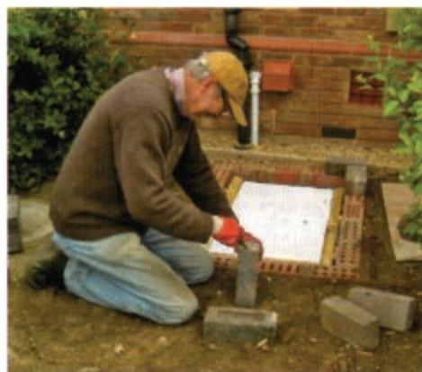
Bob working on the fat filter chamber.
