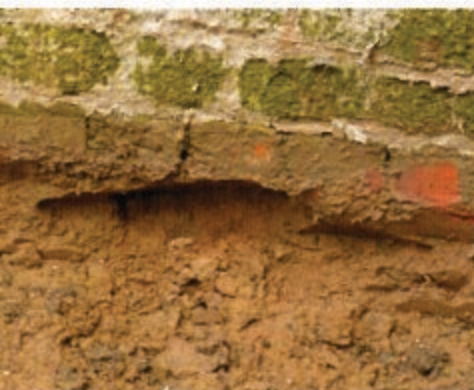
Evidence that the original structure had been built with no foundations.
