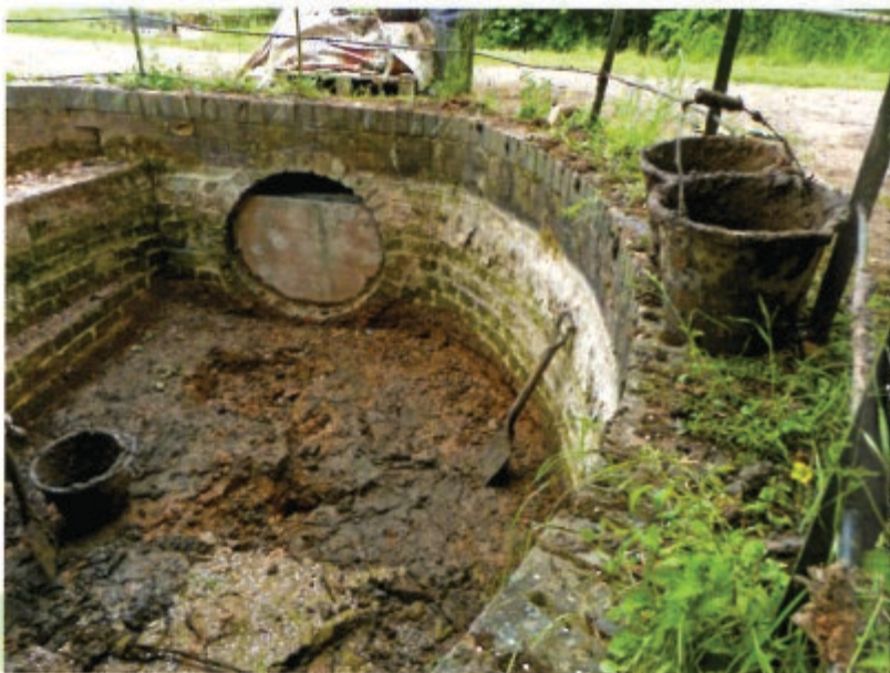
The spill weir cleared right down to its base.
