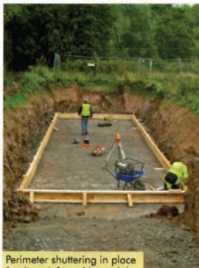
Hardcore placed on the base.
