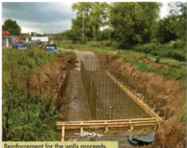
Reinforcement for the walls proceeds.
