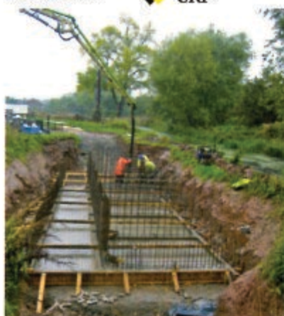
The base concrete is pumped into the foundations.
