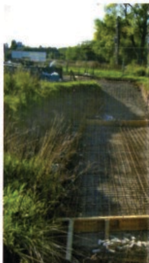
The base slab reinforcement.
