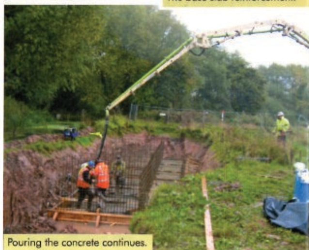
The base slab reinforcement.
