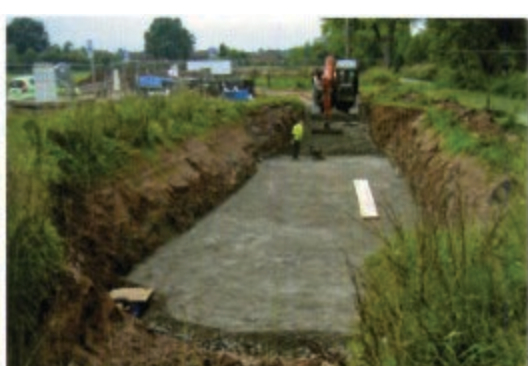
The 'blinding' concrete gives a good base to work on.
