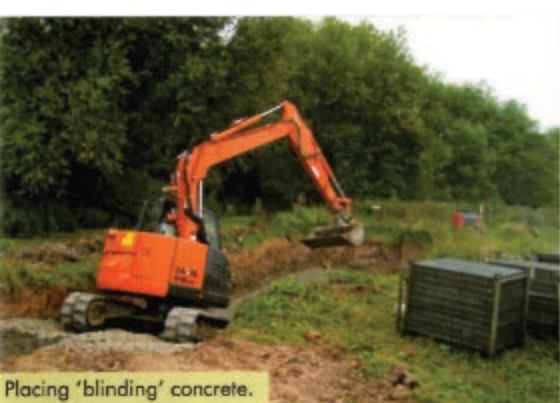
The 'blinding' concrete gives a good base to work on.
