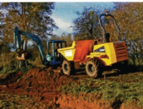
Cutting back the railway track bed to create the towpath.
