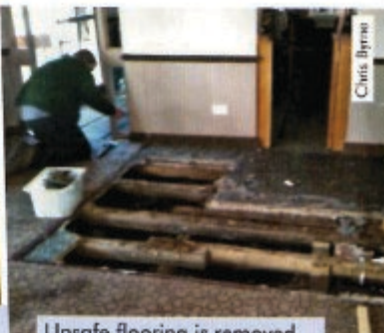
Unsafe flooring is removed prior to repair of the joists and a new floor
