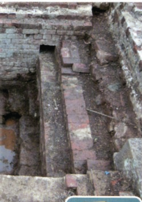
Above: Wheel and gear pit following considerable excavation.
