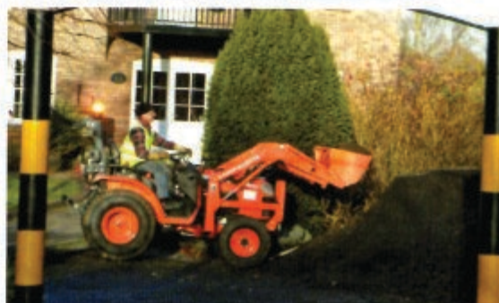
Malcolm loading road planings for car park surfacing.
