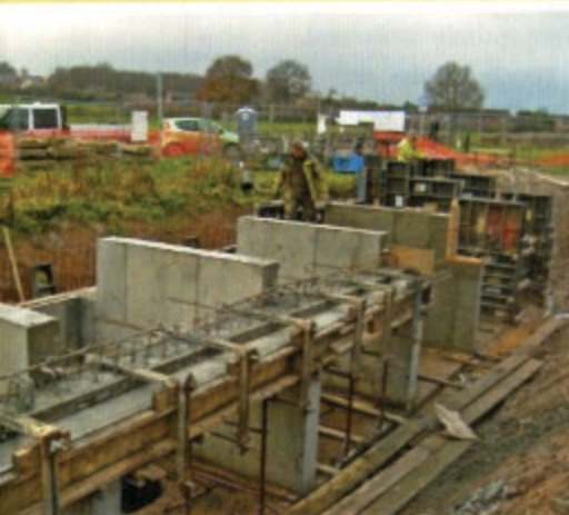
Canal-side beam to carry brick facing.
