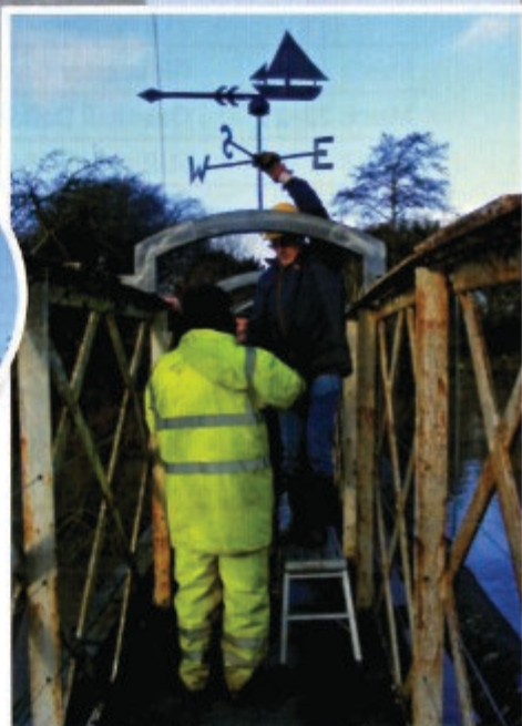
The weather vane being remounted on the bridge cross members.
