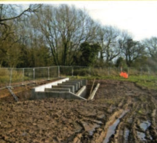
Back-filling nears completion.
