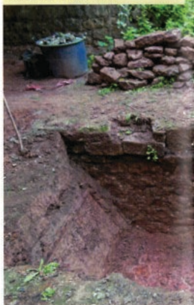
Below: Excavation of Canal at bridge. The wall is in good condition, 'rescued' displaced parapet stones are in the background.
