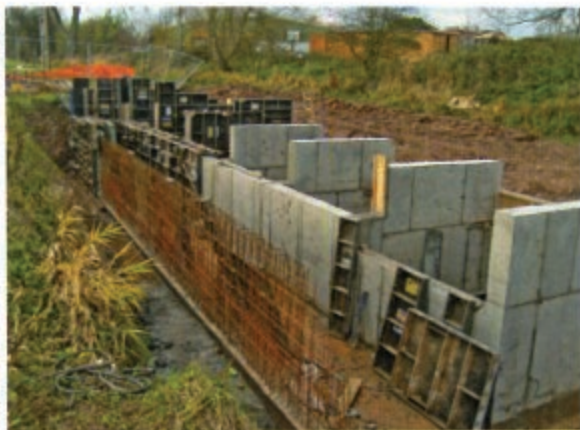
Shuttering 'struck' (removed).
