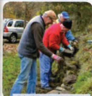
Rebuilding the dry stone wall in the car park.
