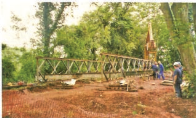
In 1997 the Bailey bridge was erected over an unstable aqueduct over Ell Brook. The restored aqueduct makes the bridge redundant.
