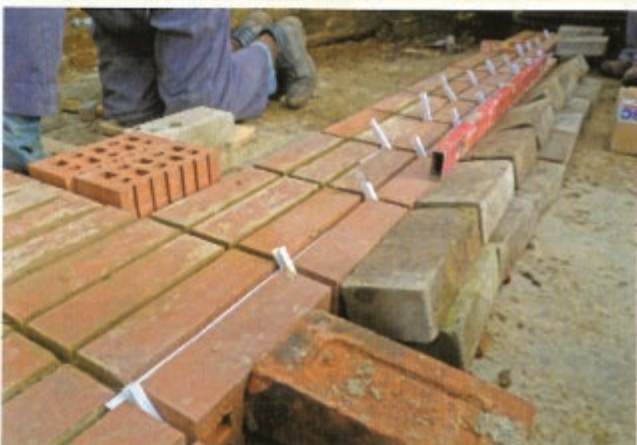
Brickwork on the weir showing the detailed work required to keep the bricks in the correct position until the mortar is set
