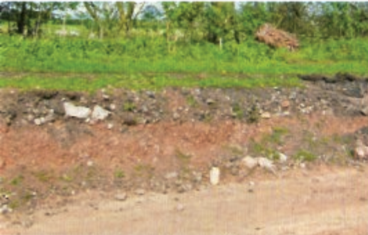
A section through the top of the railway embankment. Clay loam core with a blanket of pitching stones topped with ash and track ballast.
