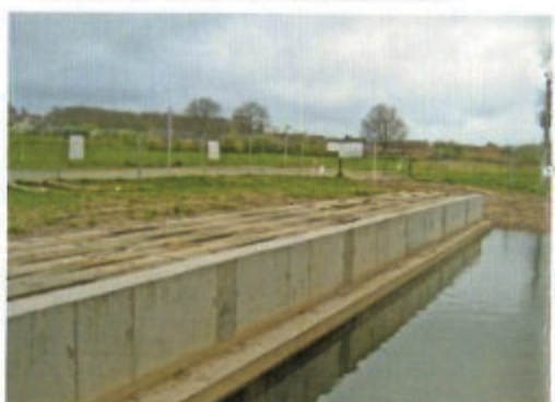
The canal side awaiting a brickwork facing.
