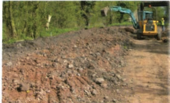
Loosening the pitching stones with quite a bit of patience and a toothed bucket on the excavator. The canal will pass through the railway bridge which can be seen in the background.
