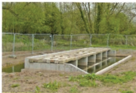
The overflow channel on the right will be dug out later.
