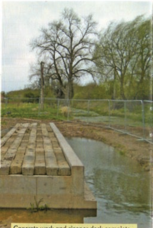
Concrete work and sleeper deck complete.
