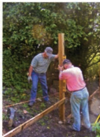
Ray checking the posts for alignment.
