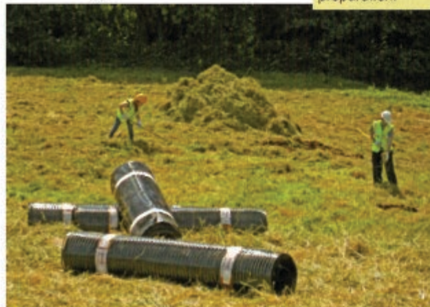
Below: Heavy rolls of geogrid are brought across the field in preparation.
