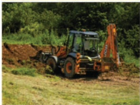
Below: Some of the earth being moved across the field in preparation for the geogrid.
