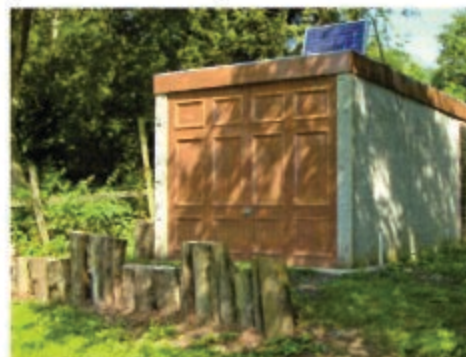
Log retaining wall in front of the site hut. Surely those logs should have been cut off level?
