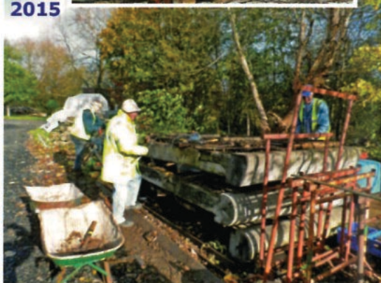
Top and above: Dismantling the lock gates.
