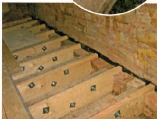
The new joists in position in one of the bedrooms.
