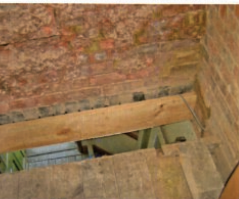
One of the new joist ends.
