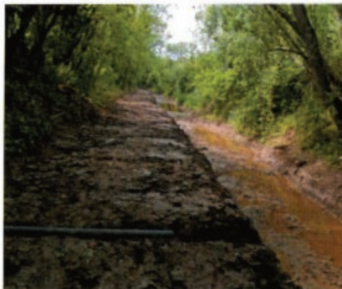
Drainage channels are laid under the towpath.
