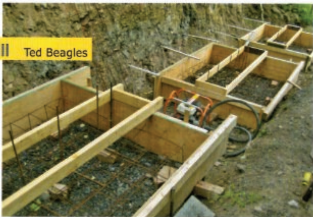
The shuttering ready for the phase one concrete pour.
