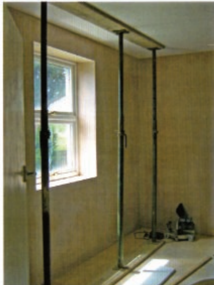
The ceiling securely propped.
