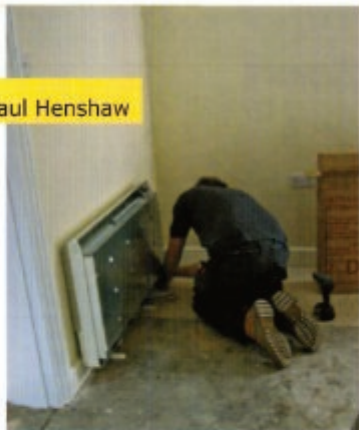
New storage heaters are fitted.
