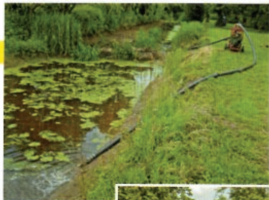
Above: The large pump in use removing water from the centre section to allow channel shaping to commence.
