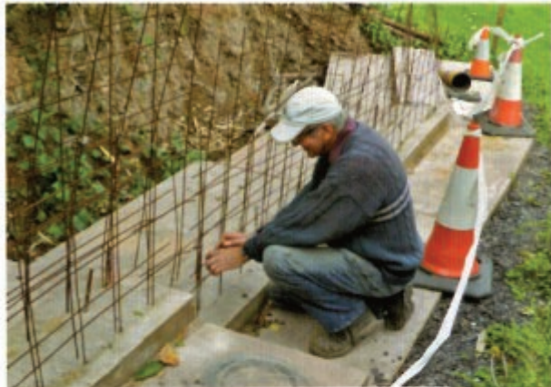
Bob erects the vertical reinforcing for the vertical concrete.
