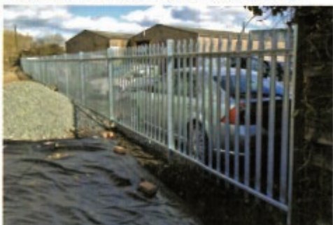
The completed palisade fencing.
