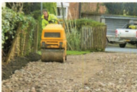
John compacting the base material.
