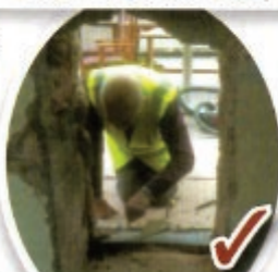
Gordon makes good the hole through the wall.
