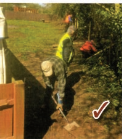
The Oxenhall team put in the fence posts for the chestnut paling.
