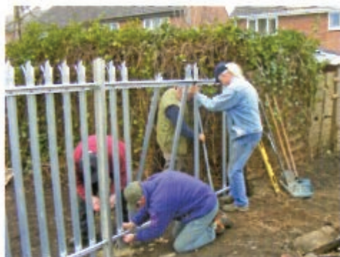
Installing final section of palisade fencing.
