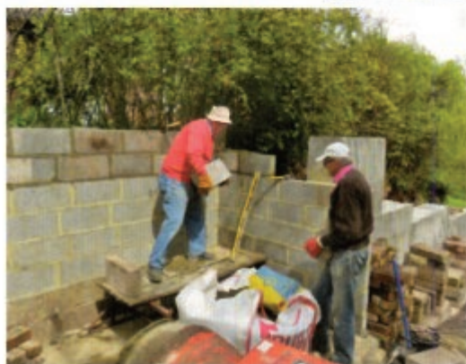
Ivor and Bob completing final the course of blockwork.
