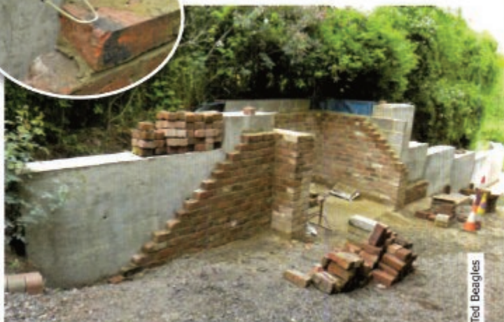
Cycle cave walls brick cladding almost completed.
