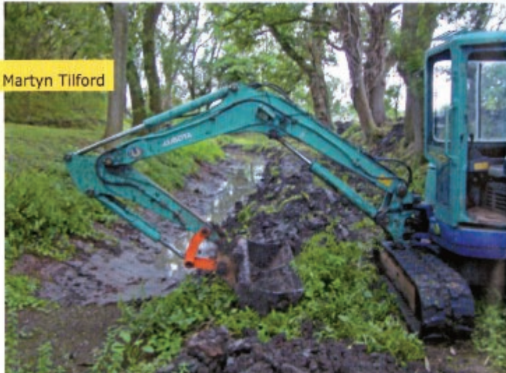
Dredging and reshaping the canal bed.
