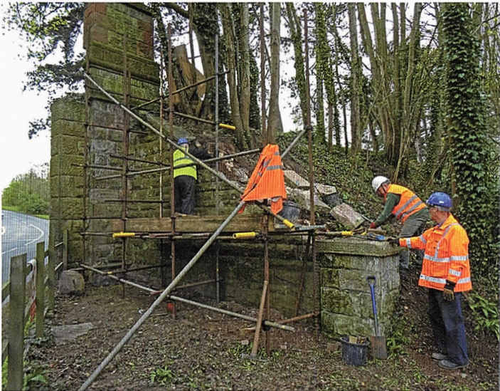
Scaffolding is erected in preparation for the repairs.
