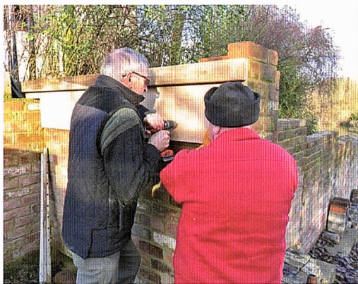
Bob and Ivor erect the L-shape shuttering.
