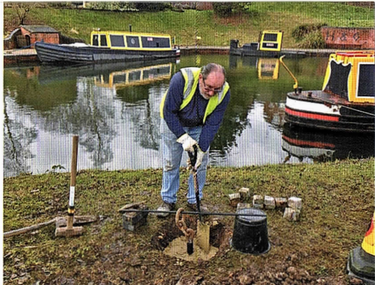
Terry repositions the mooring ring into a more convenient position.
