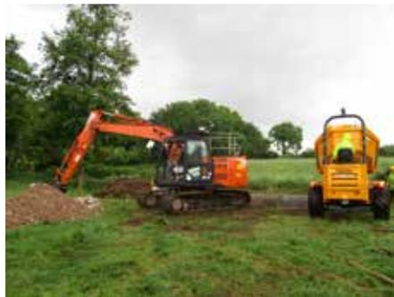
3. Infilling with crushed concrete PH
