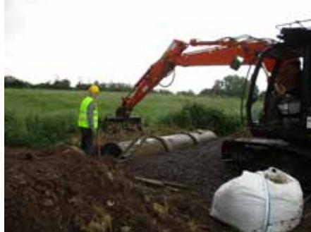
2. Lowering the pipes into the stream bed PH
