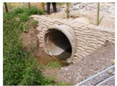
5. The head wall under construction AM
