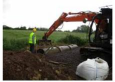
2. Lowering the pipes into the stream bed PH
