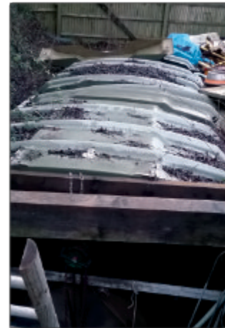
The biodisc unit with distressed 80mm driveshaft and drive train removed and the drive train ready for refitting.
